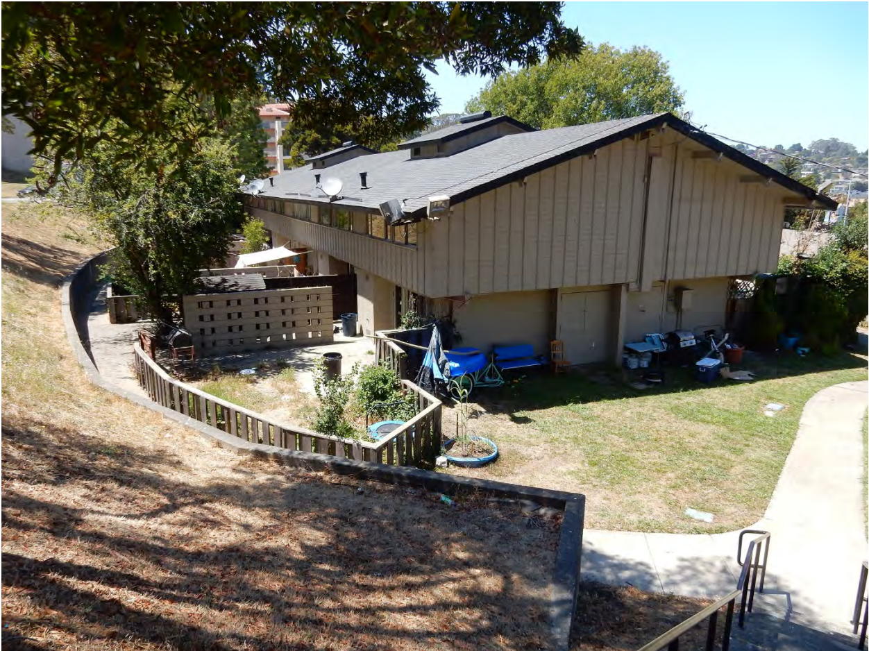
One of the two-story low-rise residential buildings. Each unit was on two levels with exposed beam ceilings, and each unit had its own outdoor terrace. Buildings were set on level pads graded into sloping sites. (Douglas Nelson photographer, July 23, 2021)
