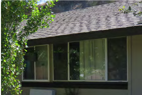
Typical 2- and 3-lite sliding windows of Type C buildings (251-57 Drake Ave)
