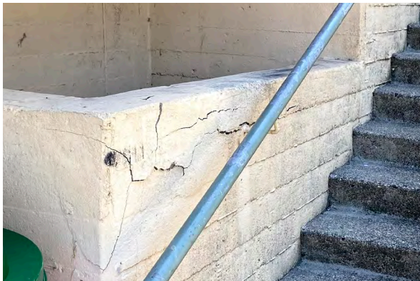
Cracks and patch failure (Type A - 89 Cole Drive)
