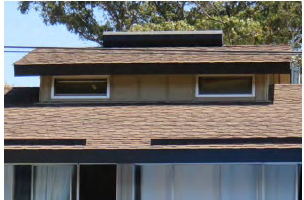
Typical awning windows at Type B buildings (161-75 Drake Ave)
