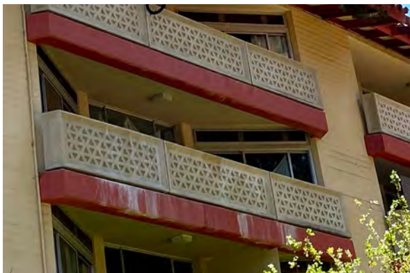
White stains at the balconies (Type A - 79 Cole Drive)
