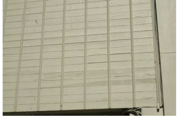
Typical redwood siding with battens at Type B and AOMB buildings (Type B - 62-76 Cole Drive)
