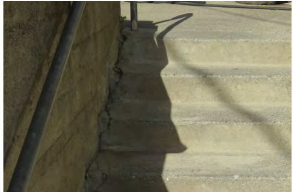
Corner crack at concrete steps
