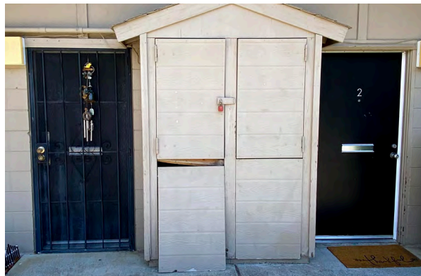
Typical wood flush doors with (left) and without (right) security doors at Type E buildings; note mail slots (2-8 Cole Drive)
