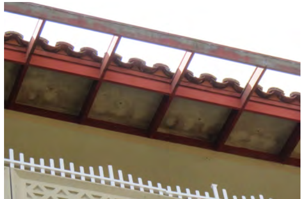
Typical staining on the clay tile roof soffit boards, likely from water damage (Type A - 419 Drake Ave)
