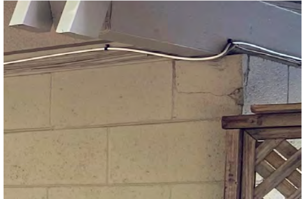
Cracked and spalled CMU unit (Type C - 341-47 Drake Ave)
