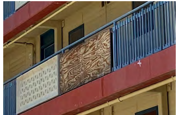
Plywood infill and steel railings at an access gallery
