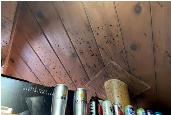
Staining on the ceiling of a Type E apartment, likely from the kitchen grease.
