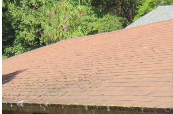
Slope of the AOMB roof distorted where modified to accommodate the new addition on the western end
