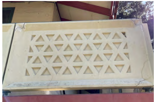
Cracks and spalls in precast concrete screen; note small insect nest at the top-right corner (Type A - 49 Cole Drive)
