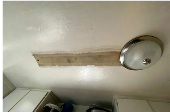
Typical plastered concrete ceiling in Type A buildings
