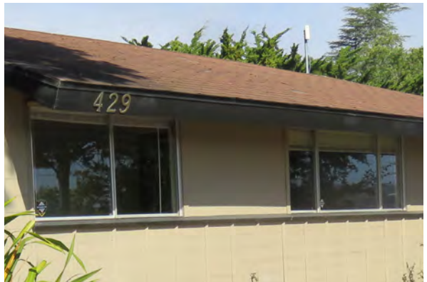
Typical 2- and 3-lite sliding windows of AOMB
