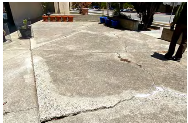
Cracked and displaced concrete slab
