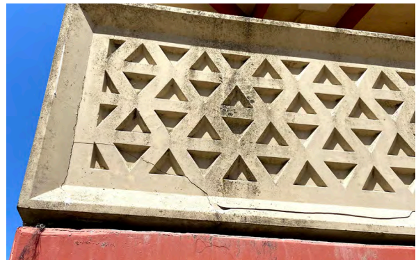
Crack in precast concrete screen (Type A - 69 Cole Drive)
