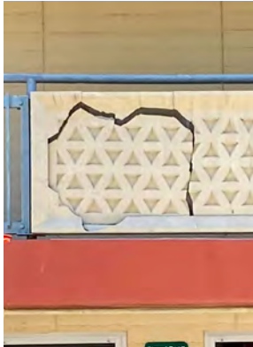
Composite panel failure (Type A - 79 Cole Drive)
