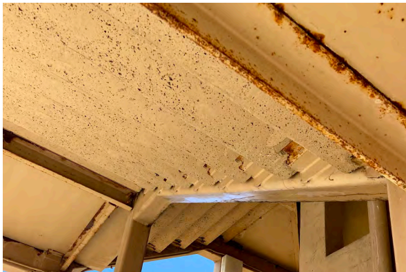
Typical corrosion and paint deterioration at steel-frame staircases of Type A buildings
