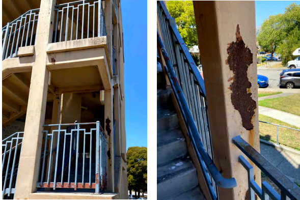
Typical corrosion and paint deterioration at steel-frame staircases (Type A - 79 Cole Drive)
