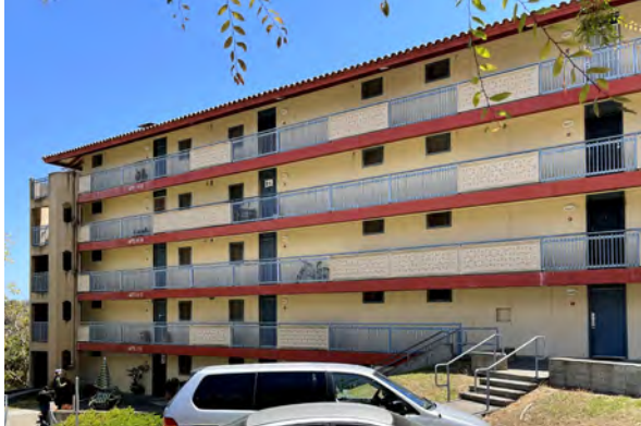
Precast concrete screens, metal railings, and handrails at a Type A building (409 Drake Ave)
