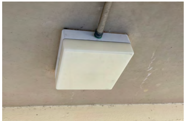
Typical ceiling-mounted square light fixture
