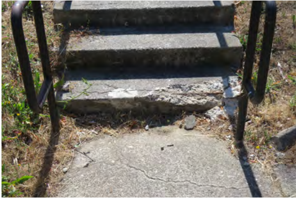
Concrete cracks and spalls and exposed corroded rebar at a staircase
