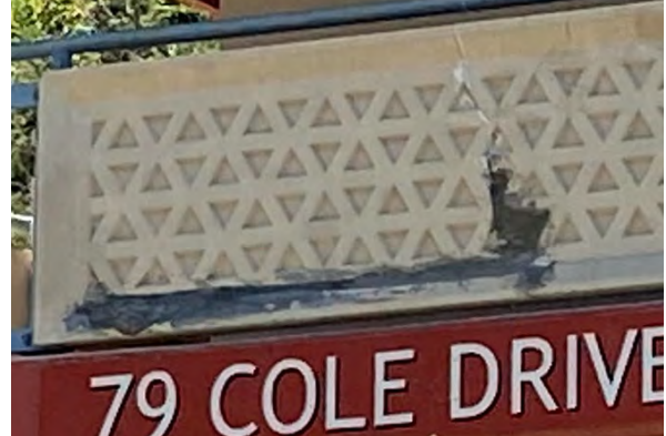
Incompatible patch repair at a composite panel (Type A - 79 Cole Drive)
