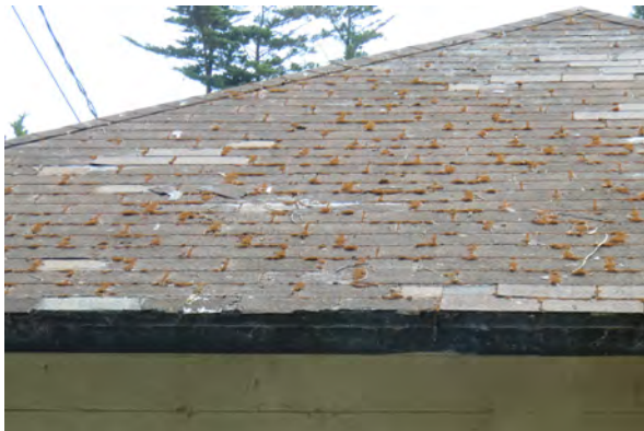
AOMB roof exhibiting cracked, detached, and missing shingles and biological growth
