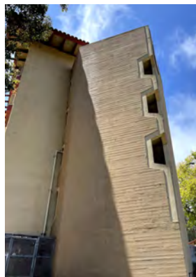
Hexagonal openings in the Type A stairwell walls (left); non-original rectangular and hexagonal openings (right)
