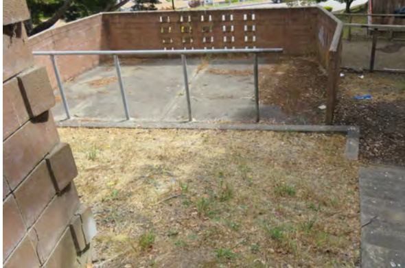
CMU block fence exhibiting cracks, soiling, and biological growth (Type A - 419 Drake Ave)
