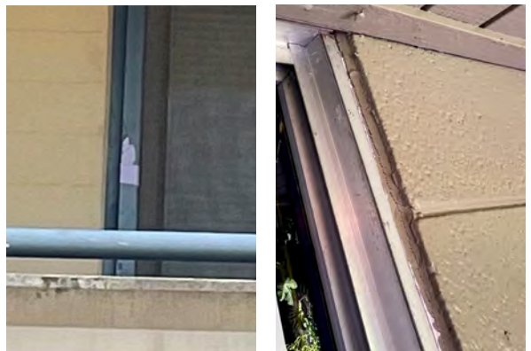
Example of paint deterioration and deteriorated perimeter sealant
