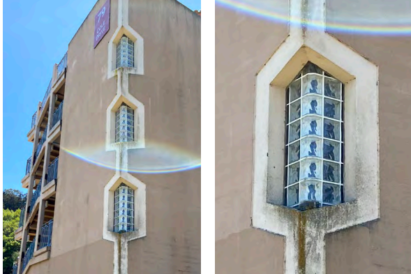
Typical glass block infill modification of the original design at hexagonal openings (Type A - 79 Cole Drive)
