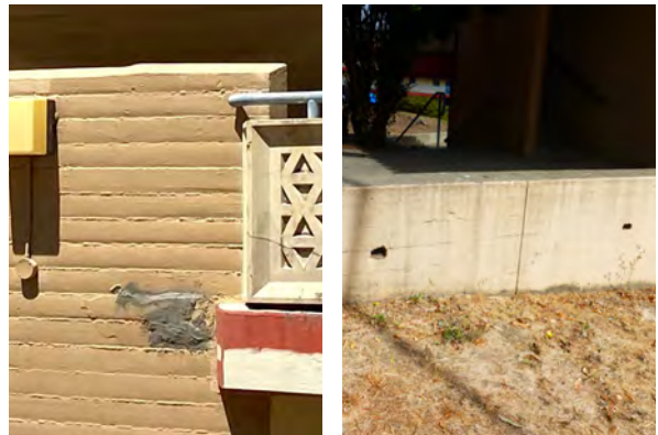
Non-matching patch (Type A - 79 Cole Drive) (left); large holes in a retaining wall (right)
