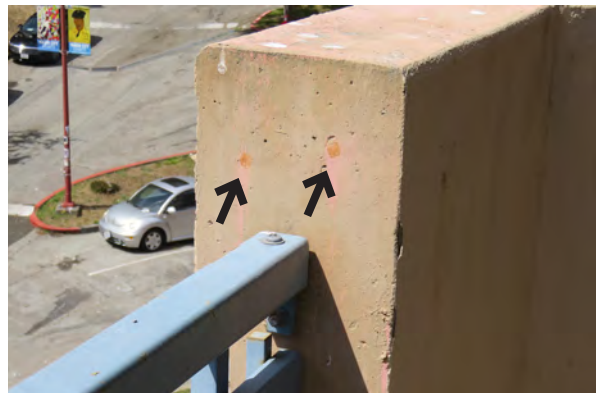
Mild corrosion at exposed rebar in the concrete walls (Type A - 419 Drake Avenue)
