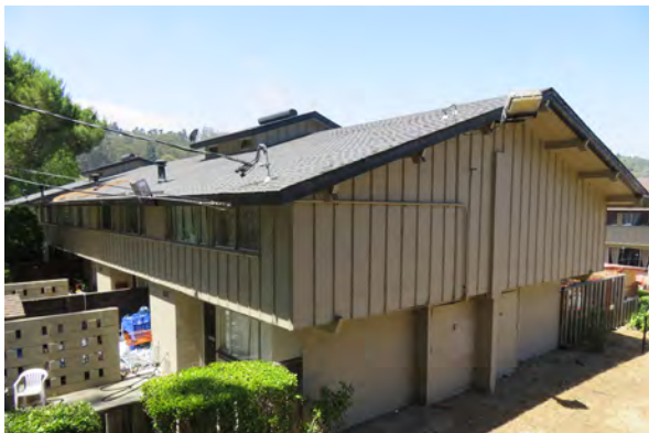
Type B building (141-55 Drake Ave); note CMU block wall and horizontal redwood siding with vertical battens
