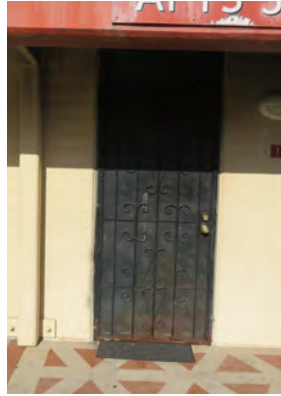
Metal security door (Type A - 59 Cole Drive)
