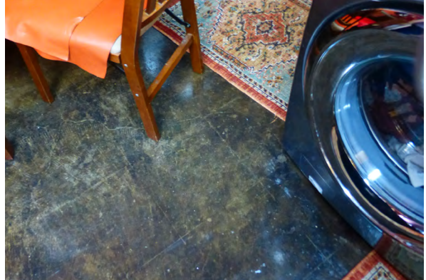
Uncovered concrete floor in a Type C kitchen after resilient tile removal
