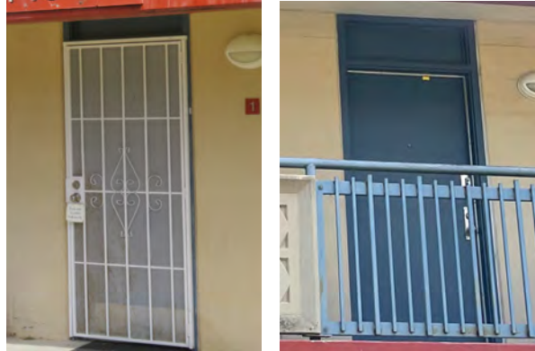
Typical wood flush doors with transom, with security door at Type A buildings (left) and without security door (right)
