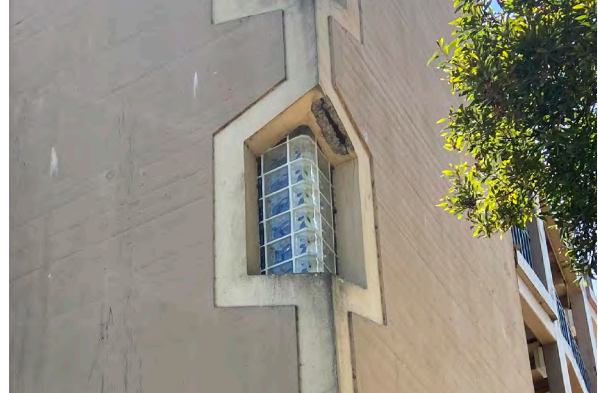
Spalled concrete at a hexagonal stairwell opening (Type A - 69 Cole Drive)
