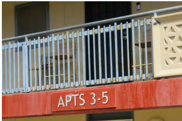
Steel railings exhibiting corrosion and paint deterioration
