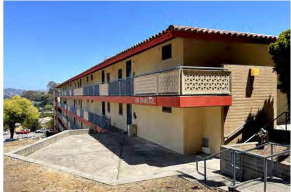
Figure 14. Pentagon-shaped terrace with seat walls, and concrete stair with metal pipe railing
