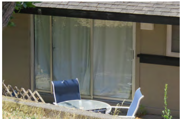
Typical 3-lite aluminum sliding doors at Type C and E buildings (Type E - 21-27 Cole Drive)
