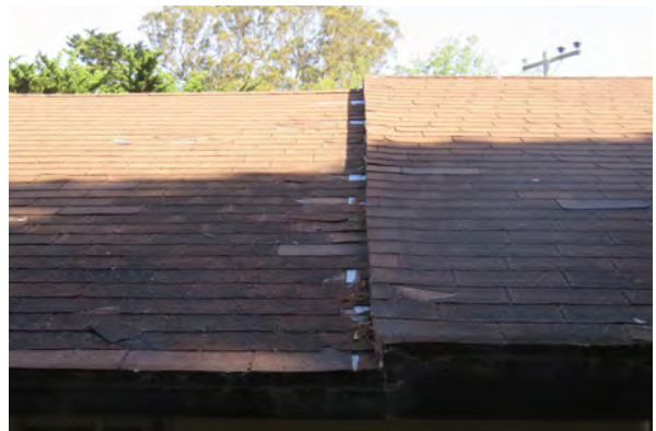
AOMB roof exhibiting cracked, detached, and missing shingles
