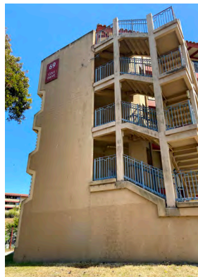
New exposed steel and concrete staircase added to Type A building in 2002 (69 Cole Drive)
