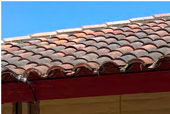
Typical soiling and biological growth on the clay tile roofs of the Type A buildings (79 Cole Drive)
