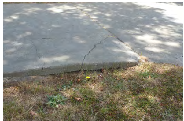
Cracked and displaced concrete slab
