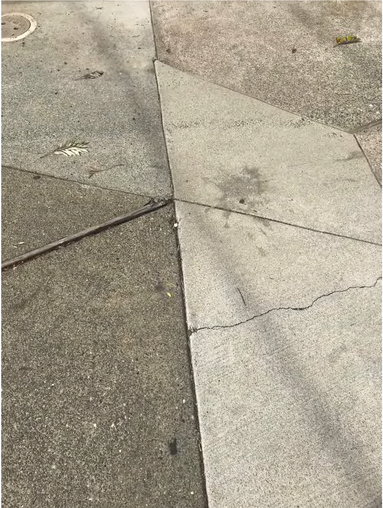
Deteriorated paving, original and replacement
