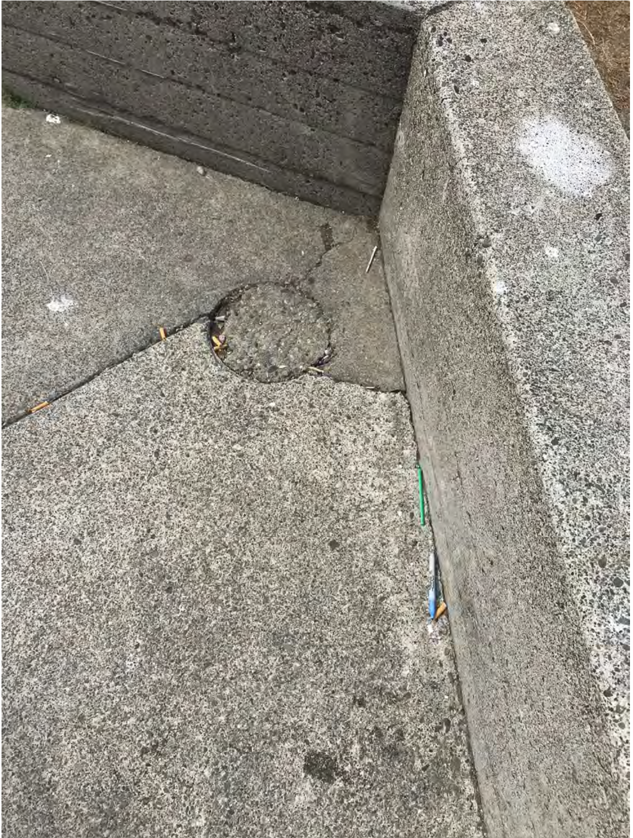
Drain filled with concrete
