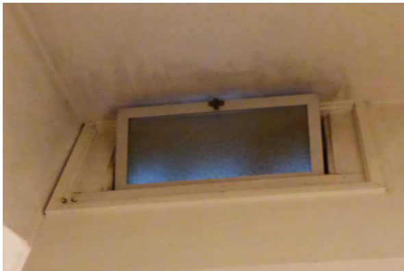
Typical hopper window in a Type E apartment bathroom
