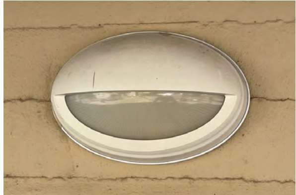
Typical wall-mounted rounded hood light fixture
