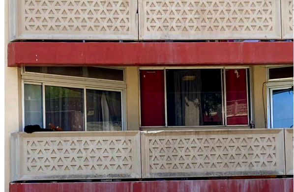
Cracks and spalls in precast concrete screens (Type A - 99 Cole Drive)
